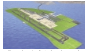
The cutting-edge Chubu Centrair International Airport functions 24 hours a day.
