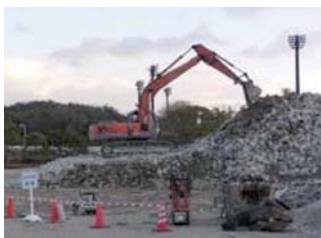
Concrete mass being recycled
