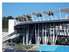
Supports with steel-rake structure
