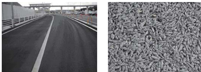
Waste tire pavement and a magnified view
