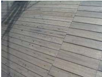
Thinned wood on the Loop: Left part is made from thinned wood of cedar produced in Aichi Prefecture
